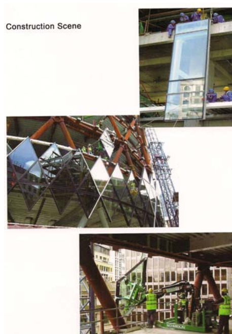
Figure 3. Installation of SunGroup thin-film PV panels
